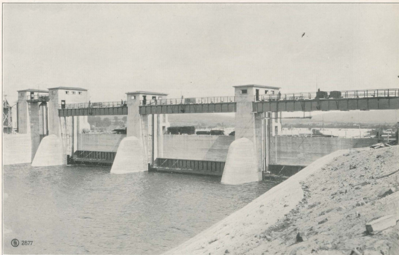
General view of Weir and Intake Bu
