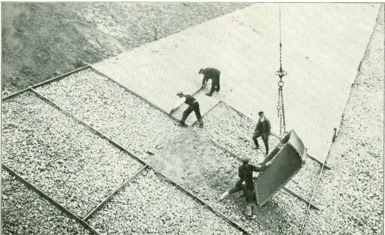
Concreting of slab on the slopes
