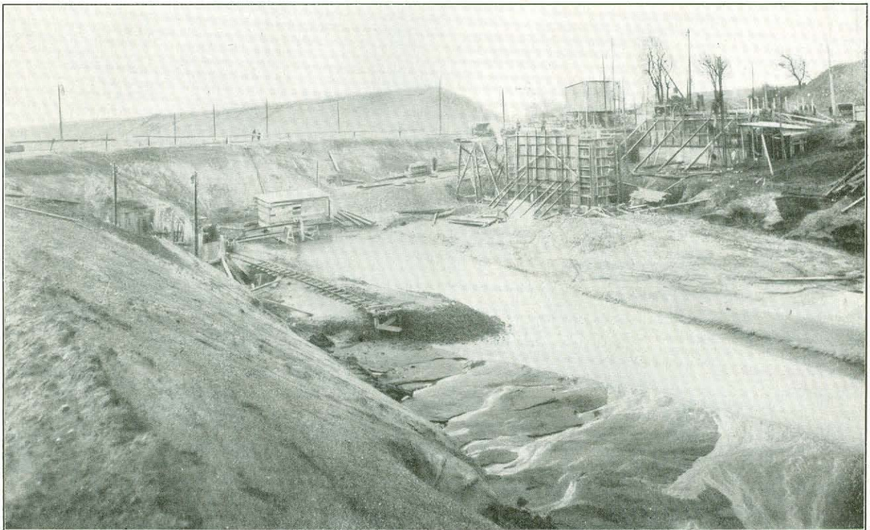
Excavation of foundation and concreting of the piers and abutments
