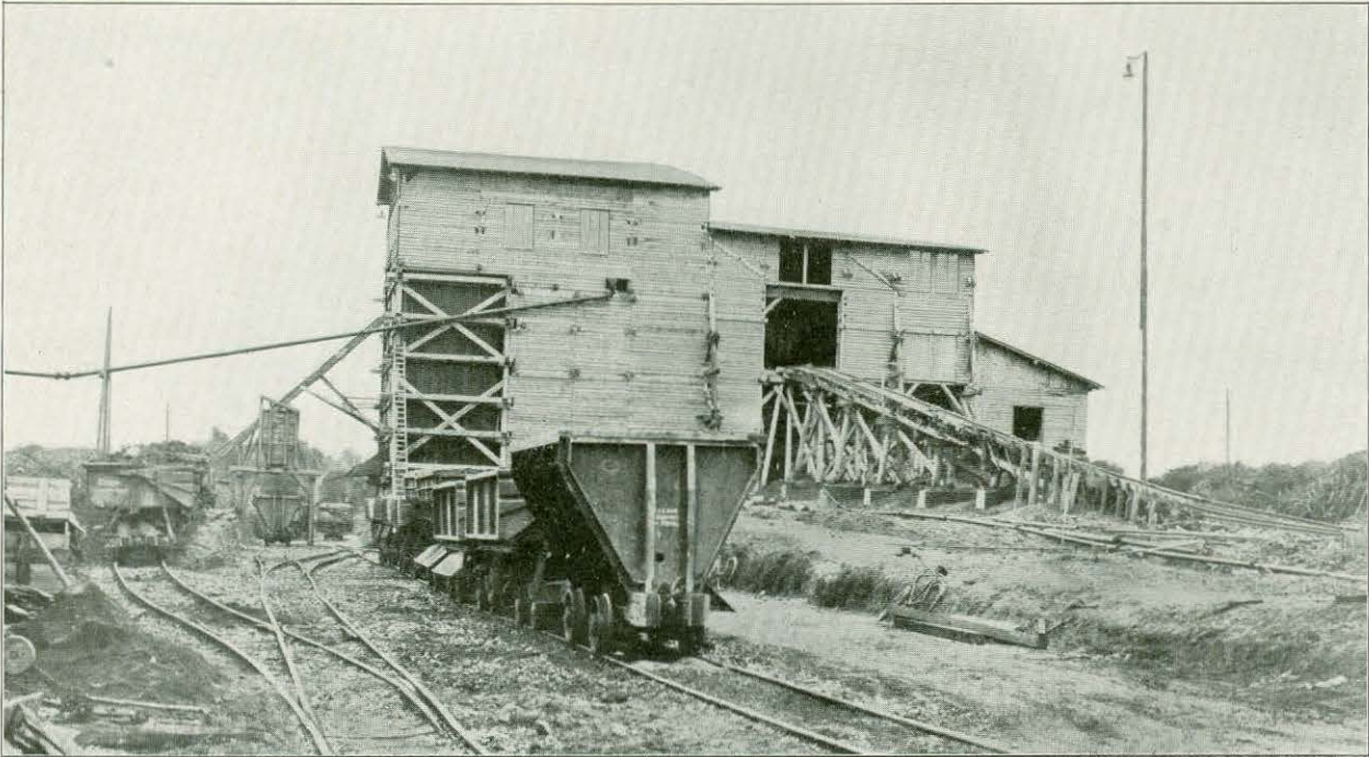
Stone Crushing and Washing Plant at Clonlara
