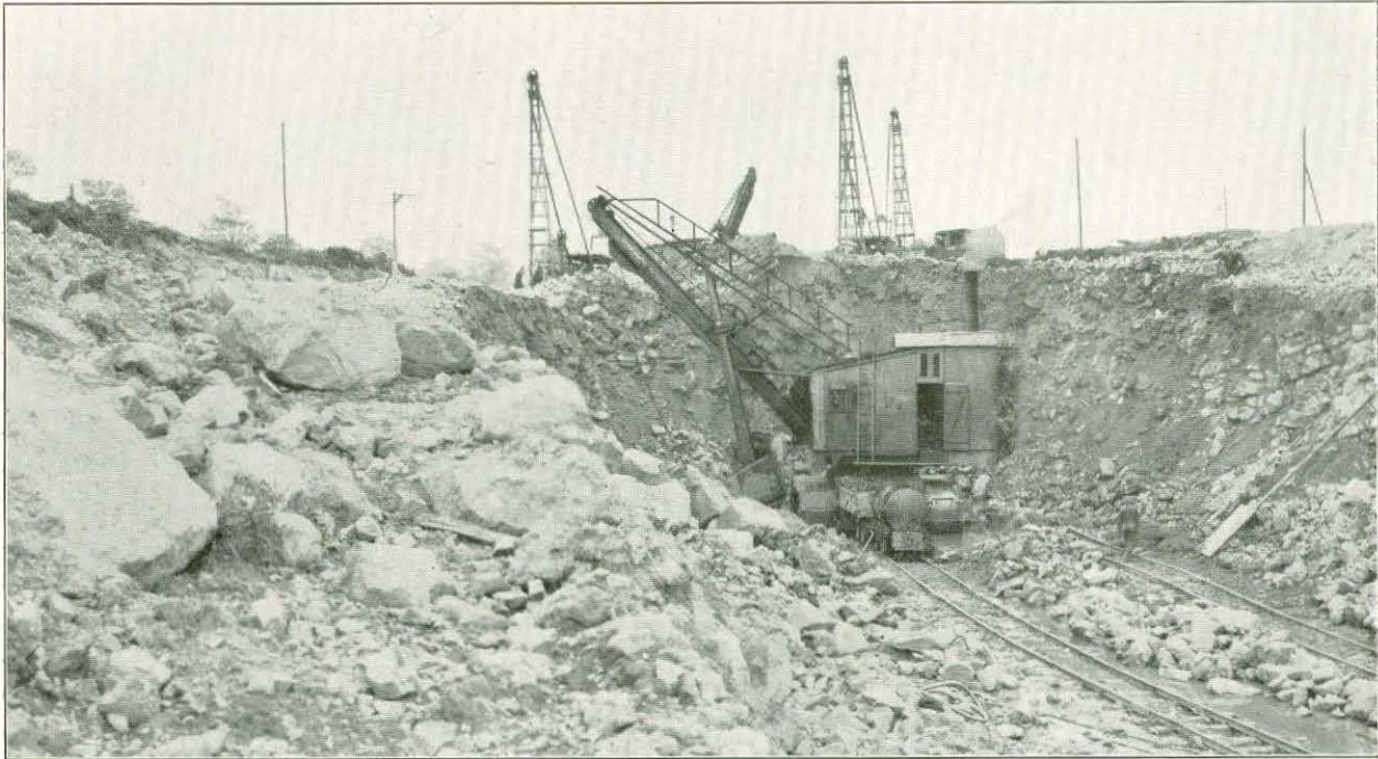
Shovel excavators and boring machines in the Tail Race
