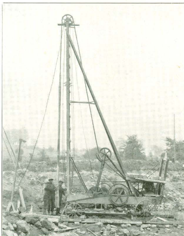
Boring machine with drop hammer
