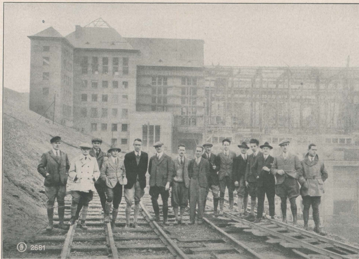
The Government and Siemens-Bauunion-Engineering staff of the Power House Building Site.
