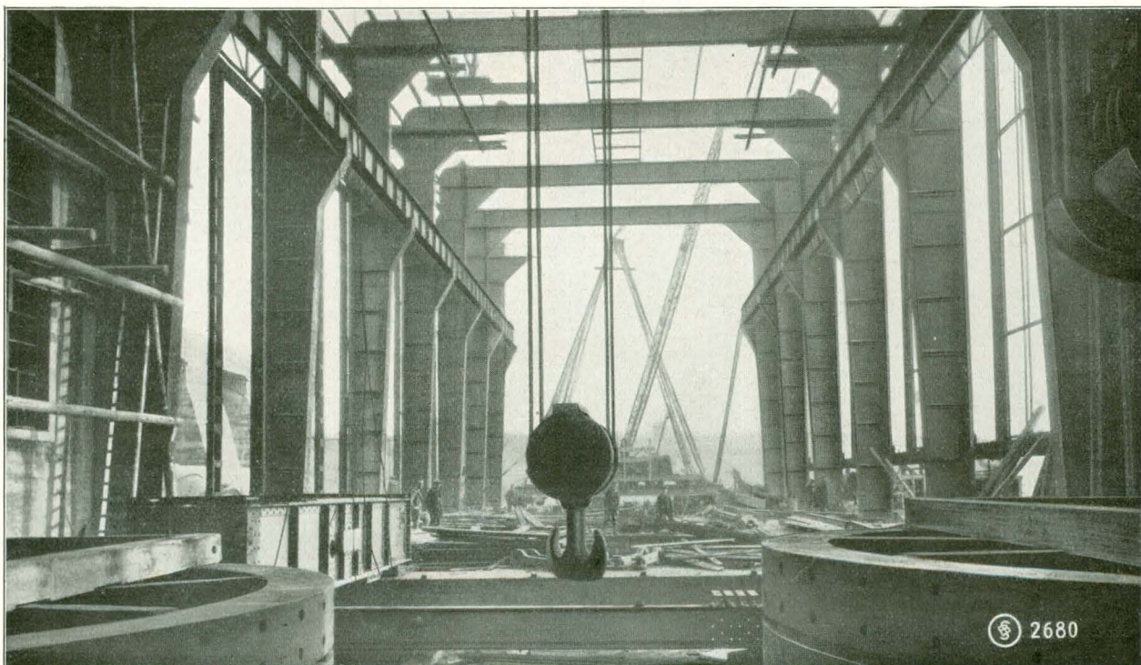
Inside view of the steel structures of the Generator Hall
