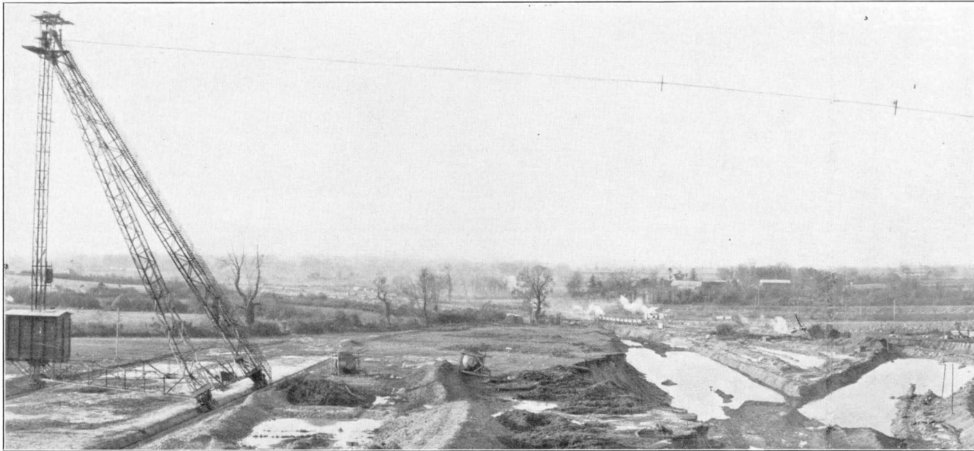
General excavation of Power Station with temporary
