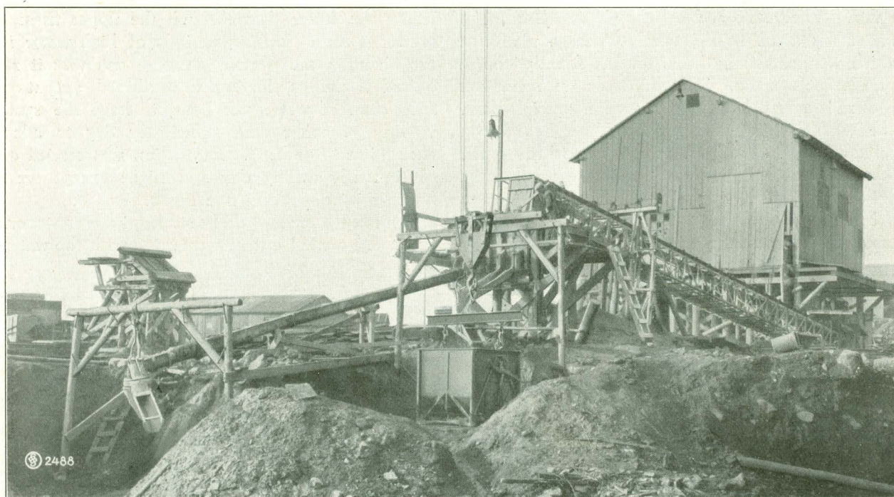
Transport of the concrete by conveyor belt to the carrier of the cable crane
