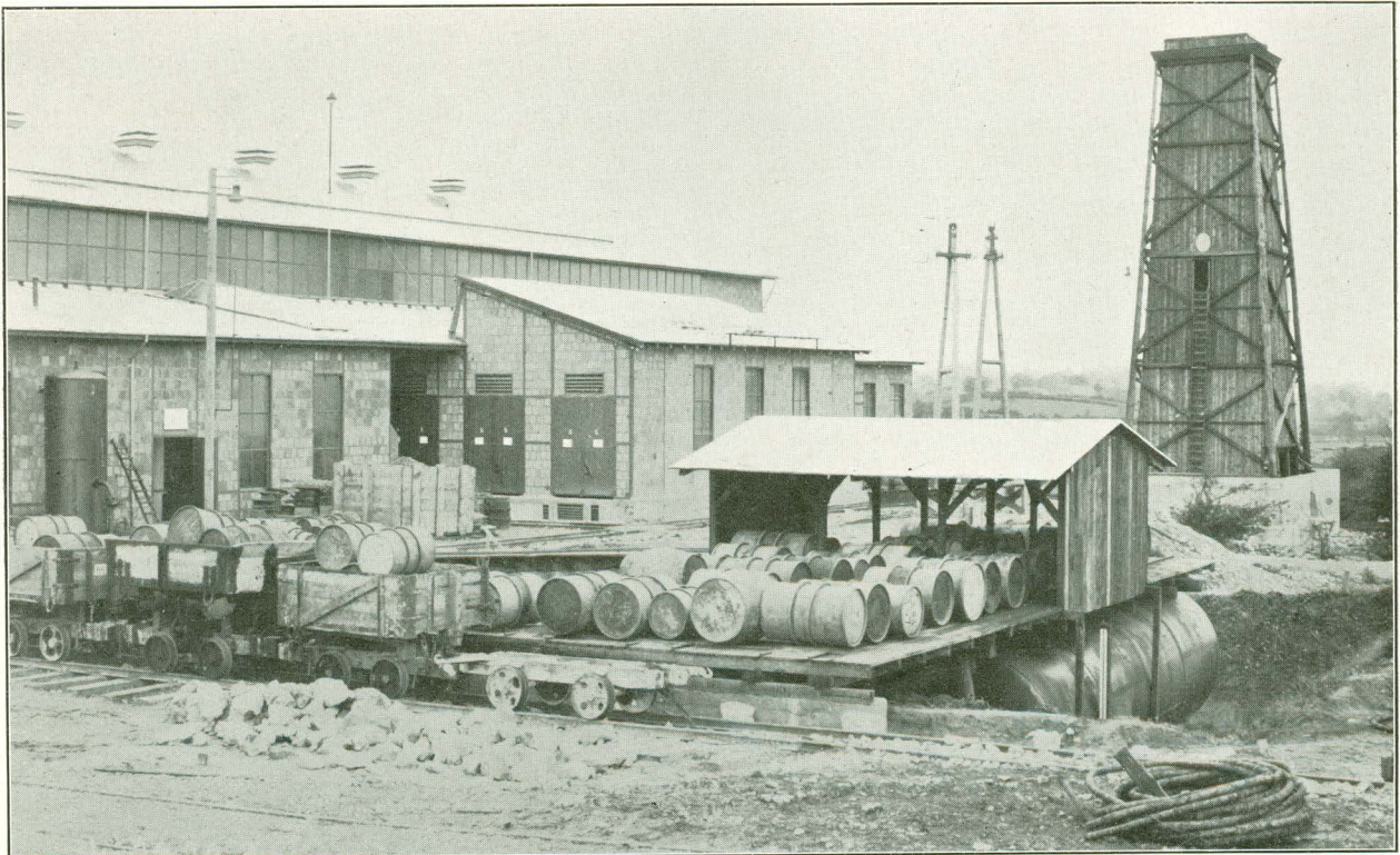
Oil Tanks for Diesel Motors of Temporary Power Station.
