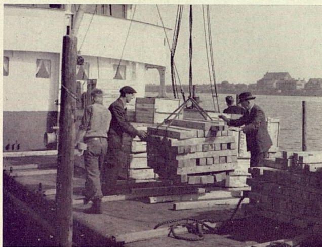
Loading supplies in Dublin on the MV 'Whitsun' for the famous beaching operation on Arranmore.
