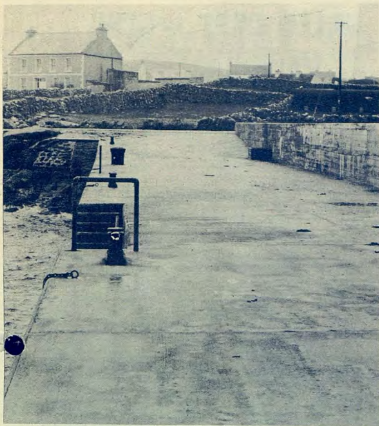
Inisheer has a pier but the C.I.E. steamer cannot come alongside.
