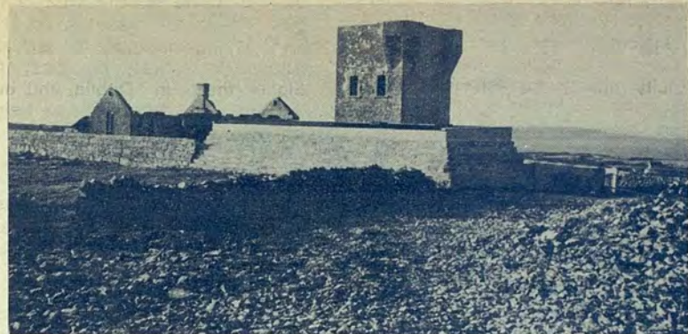
Island's water supply is pumped from a pump house to this reservoir and gravity fed to the houses.
