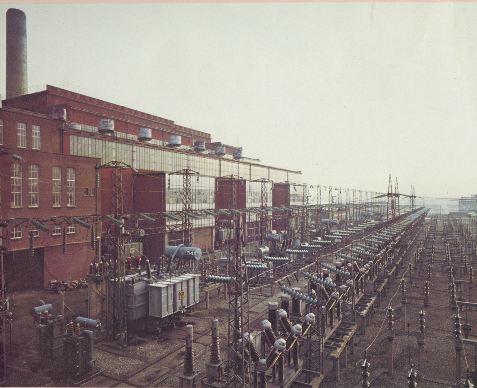
E: 110kV Compound
