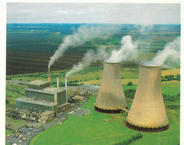
ESB Generating Station at Rhode
