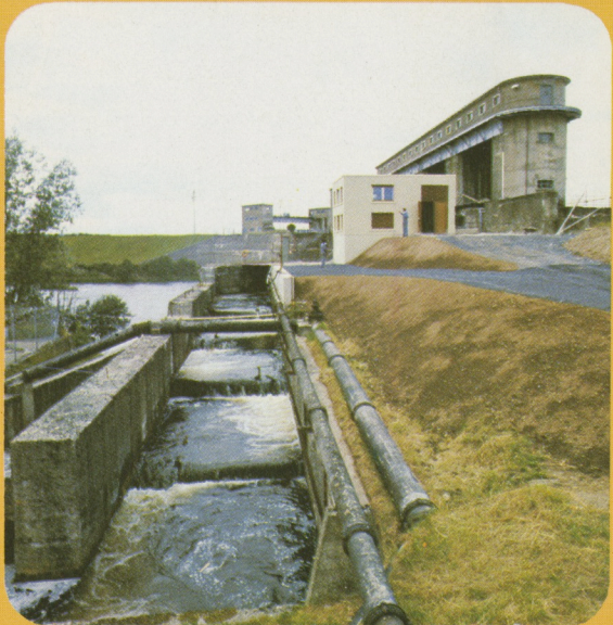
A view of the Generator House with the fish pass in the foreground.
