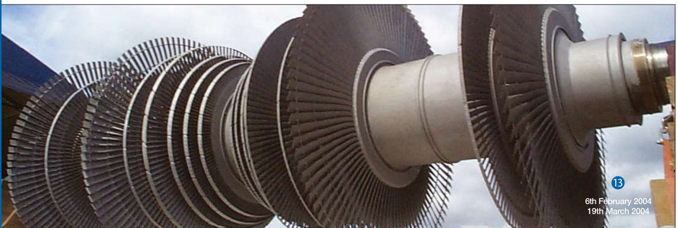
10. View of Original and New Chimney Stacks 11. Interior of Canteen 12. Generating Building 13. View of Former Turbine During Overhaul
