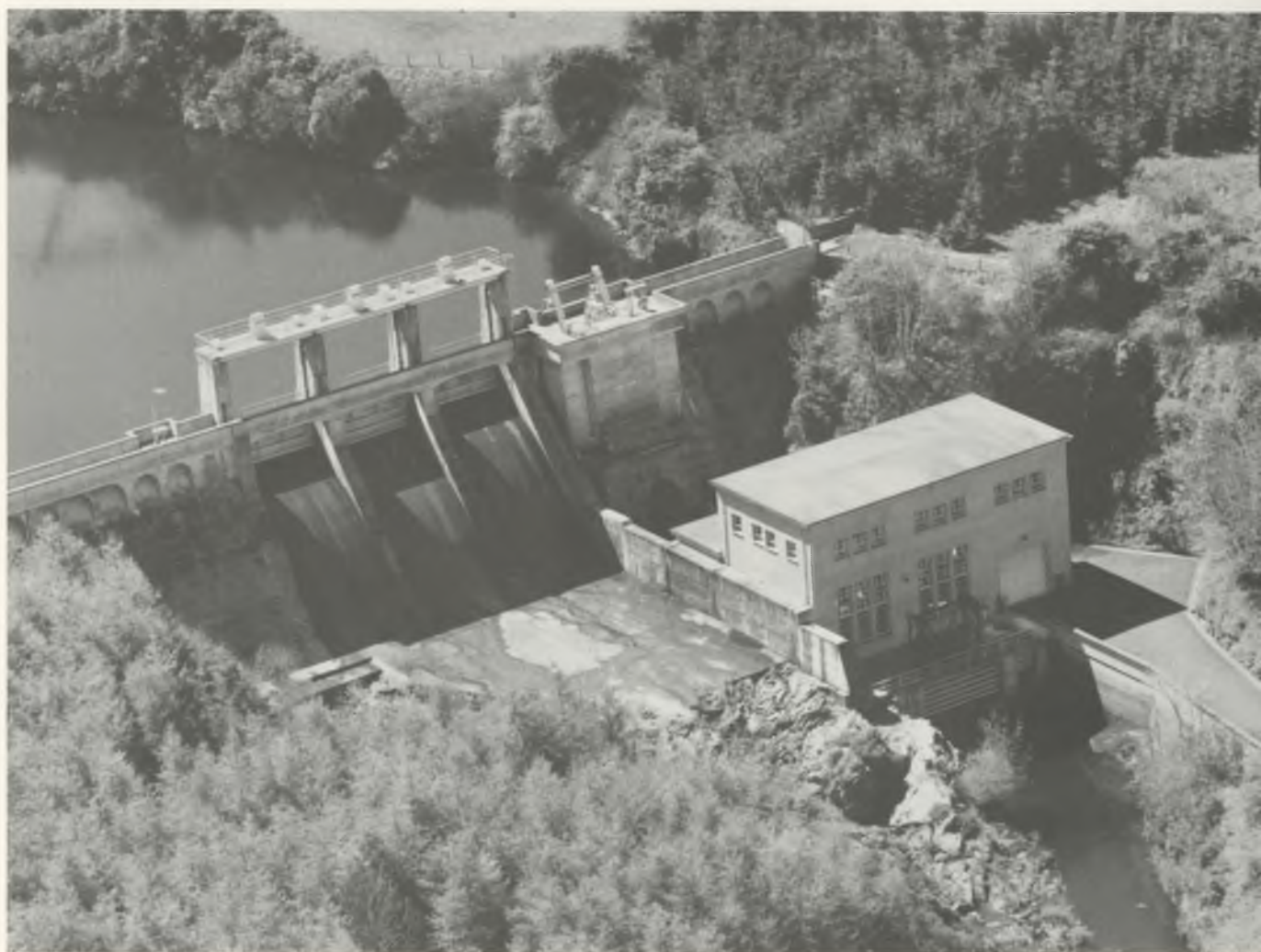
The completed power station at Golden Falls.
