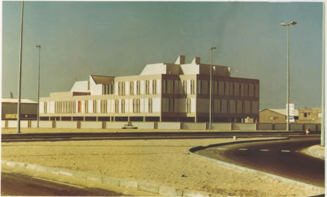
National Control Centre, Bahrain (above) Ensuring continuity of supply (left) Submarine cable crossing River Shannon (below)
