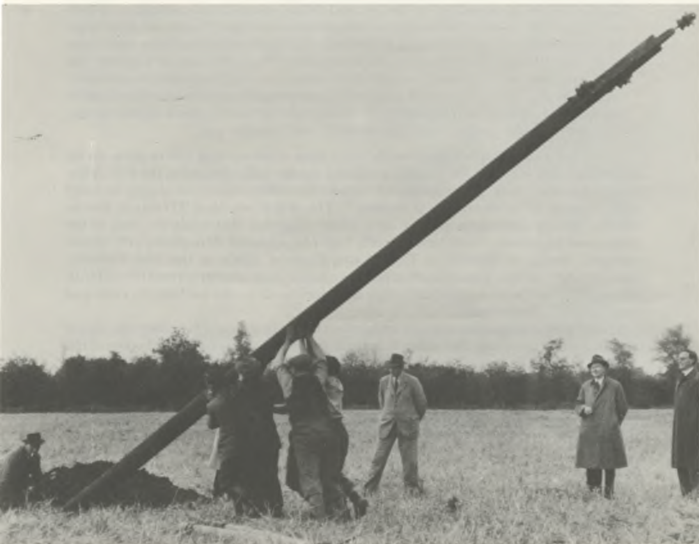
Erecting the first pole at Kilsallaghan, Co. Dublin, on 5 November 1946.
