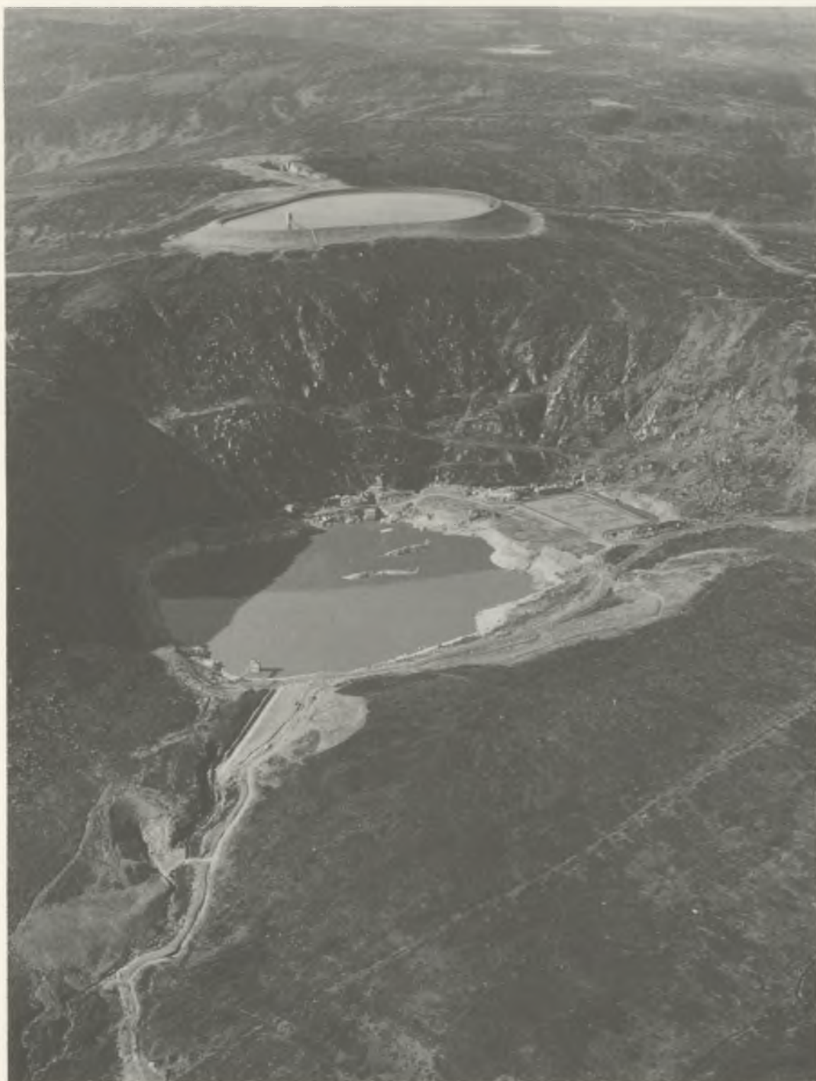
Turlough Hill: an aerial view of the upper reservoir and lower lake.
