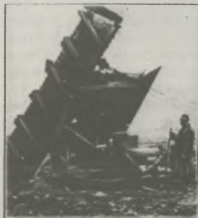
Shannon power applied to an Irish industry. An electrically operated shovel and hopper at work near Yellamore, cutting peat.
