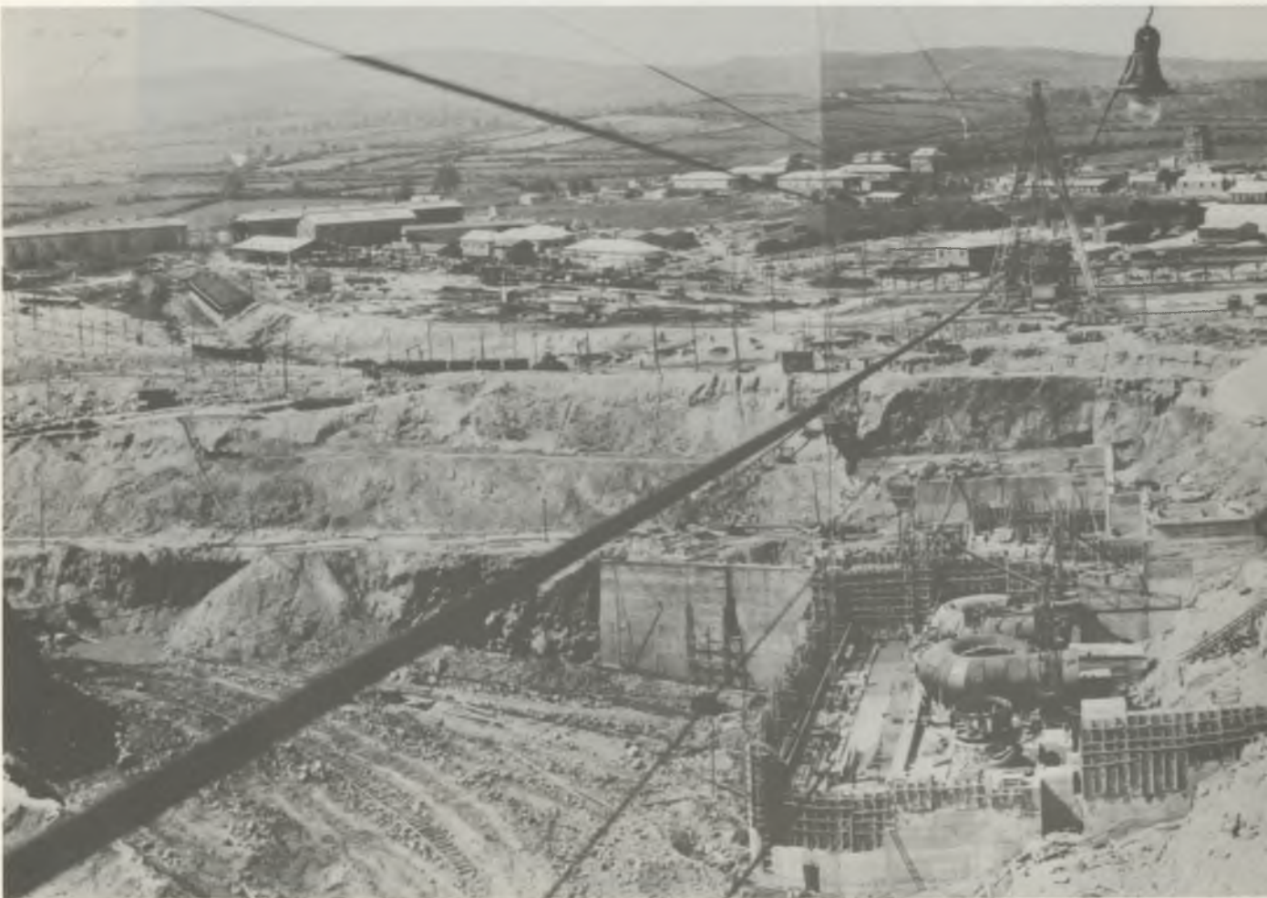
A general view of the works at Ardnacrusha.
