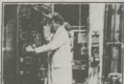
"Throwing over" the last of the main switches by which Shannon power is brought into operation. Here Daily Sketch pictures its middle pages.
